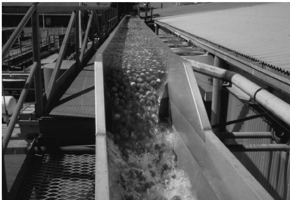
Figure 10.20 A water flume is used to convey tomatoes from the receiving area to the processing equipment.
