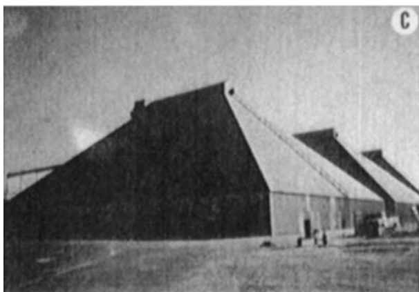
Figure 4 Cottonseed storage systems. (A) Uncovered, outside storage piles; (B) covered, outside storage piles; and (C) Muskogee buildings.
