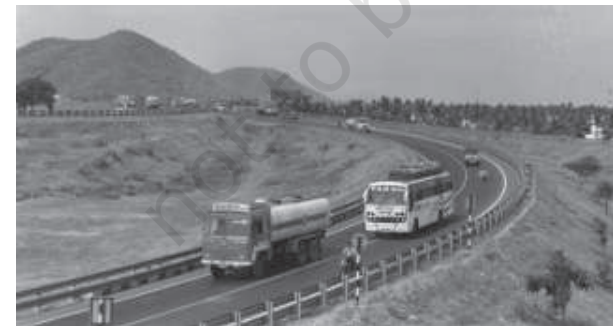
Fig. 8.1 Roads are the missing link with growth
