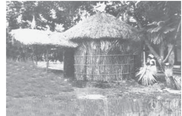
Fig. 4.2 Many poor families live in kutchha houses
