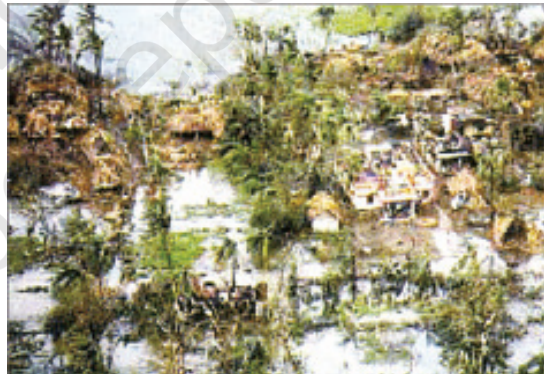
Destruction caused by a cyclone
