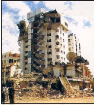
Fig. 3.3a: Destruction caused by an Earthquake in Gujarat
