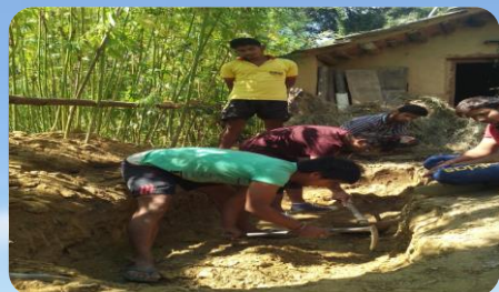
Removal of stones and gravels
