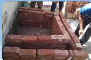
Construction of walls
