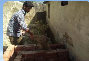
Sand and water filling in between walls
