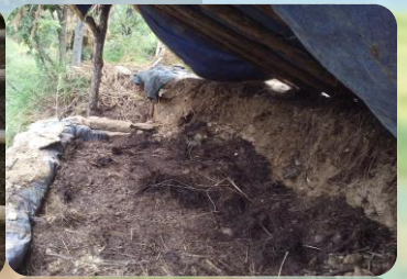
Covering of pits by canvas for protection from rainwater
