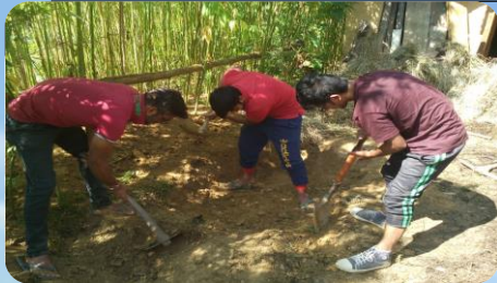
Digging of compost pit
