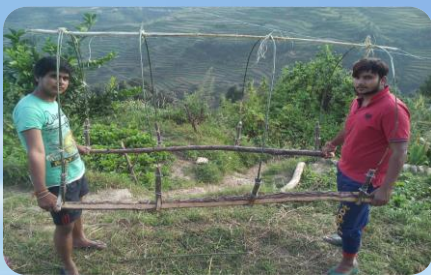
Preparing structure of Portable Polytunnel
