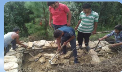
Construction of Pit walls
