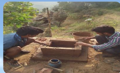
Constructing walls of mud hive
