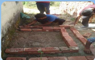
Construction of base
