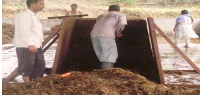
Fig. The set of a Pile former consisting of three steel boards
