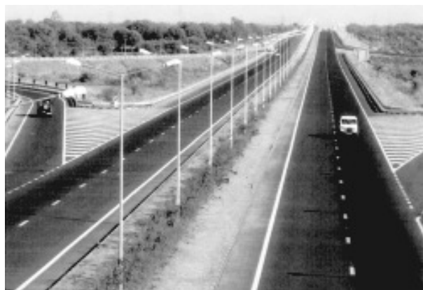
Fig.7.2: Ahmedabad- Vadodara Expressway
