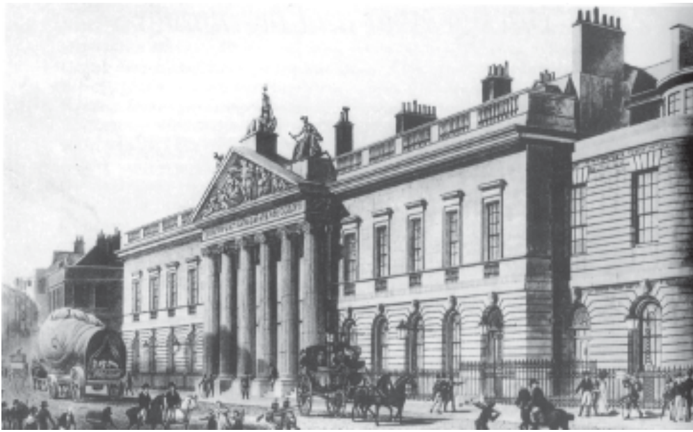
Fig. 17 – East India Company House, London.
