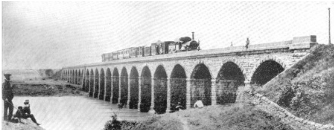
Fig. 1.4 First Railway Bridge linking Bombay with Thane, 1854
