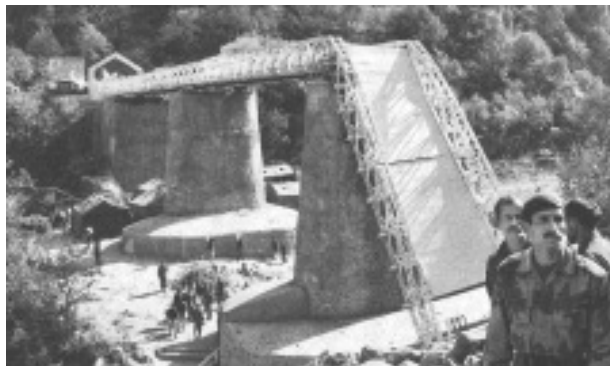
A view of the damaged Aman Setu at the LOC in Uri, due to an earthquake
