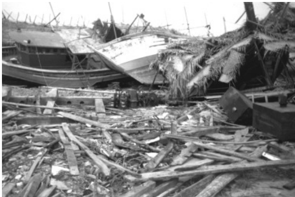
Figure 7.3 : Tsunami Affected Area
