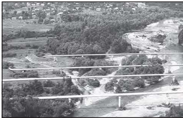
Fig. 8.17: Pipelines transporting natural gas in Ukraine
