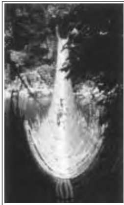
Figure 6.7 : Rope Bridge (Arunachal Pradesh)
